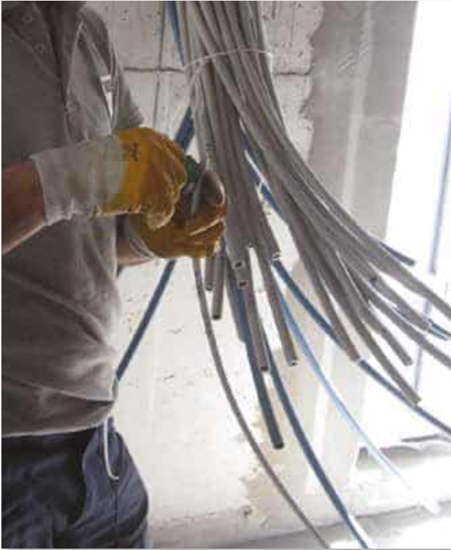
An operator stripping cables during installation.
