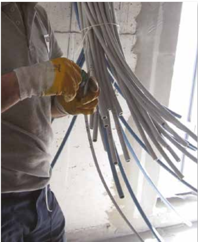
An operator stripping cables during installation.
