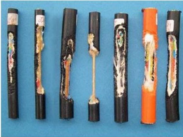
Figure 1: Cables Attacked by Rodents
