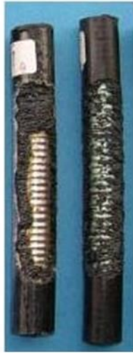
Figure 3: Armored fiber optic cable exposed to rodent attack
