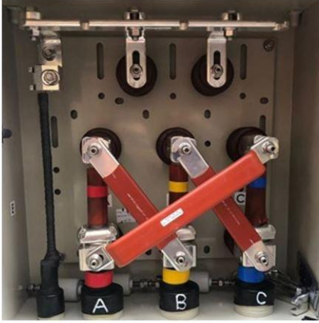
Crossover Box Connection Example
